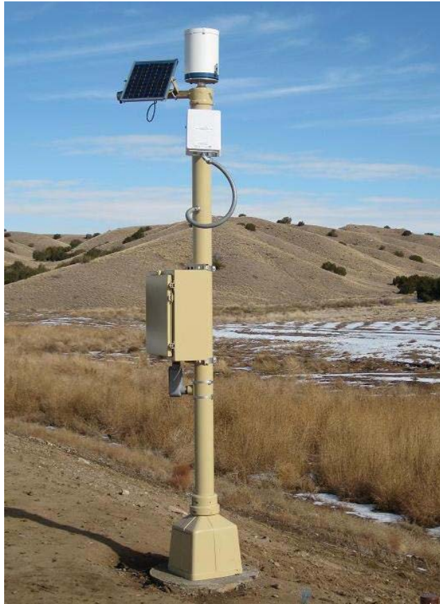
Figure 10.1 Example of a Stand-alone EWS Site (Water Tank Dam, New Mexico)
