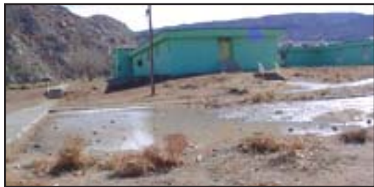
T'iis Nazbas overflow collects near a dormitory sidewalk.
