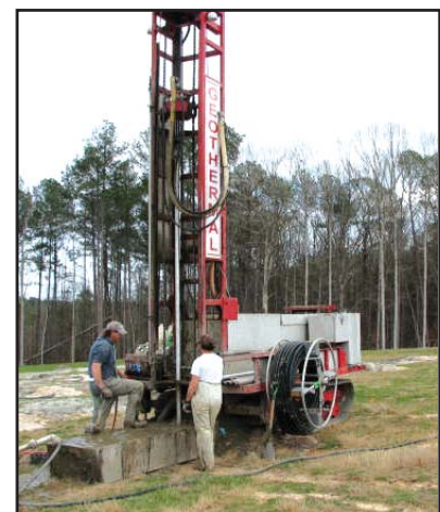
Drilling wells at Red Water site.
