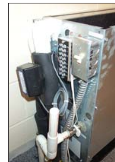
Gaining heat while underground in the earth, a water/glycol mixture is circulated by pumps (above) to a classroom heat pump (below) where it assists in heating a classroom.
