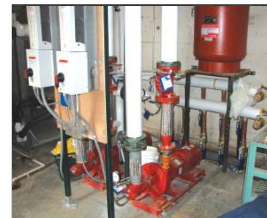
Gaining heat while underground in the earth, a water/glycol mixture is circulated by pumps (above) to a classroom heat pump (below) where it assists in heating a classroom.
