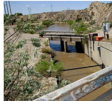
Hogback Canal is both concrete lined and unlined and serves approximately 135 miles of lateral canals
