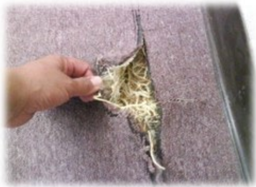
Figure 1-2. Camelthorn growing through the floors of a home on the Navajo Nation. (Photo Credit: BIA Western Navajo Agency).
