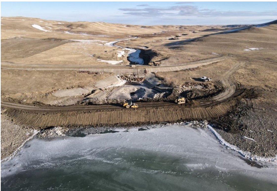
Four Horns Dam during Construction for Blackfeet Nation in Browning, MT
