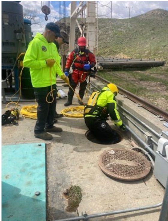
Wiota Pumping Plant at Fort Peck Indian Project, Montana – divers implementing pumps and impellers.
