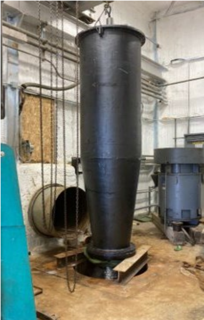
Viota Pumping Plant at Fort Peck Indian Project, Montana – reinstalling refurbished pump and housing.
