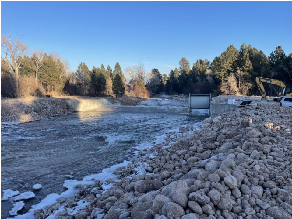
Uintah River bifurcation replacement, Uintah Indian Irrigation Project, Utah – construction complete
