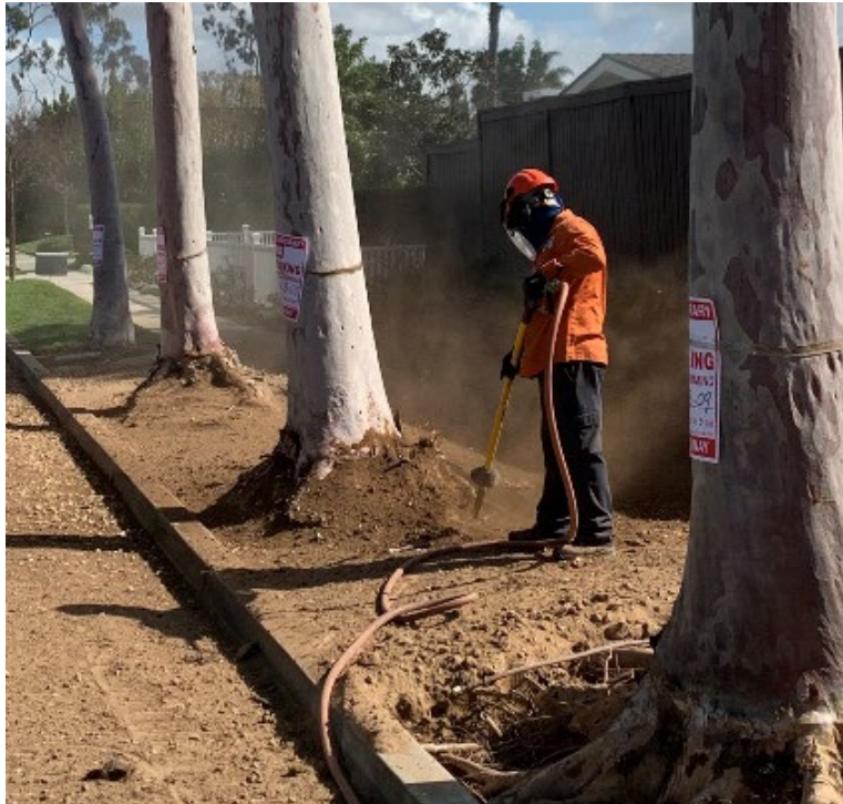
Clearing roots for assessment
