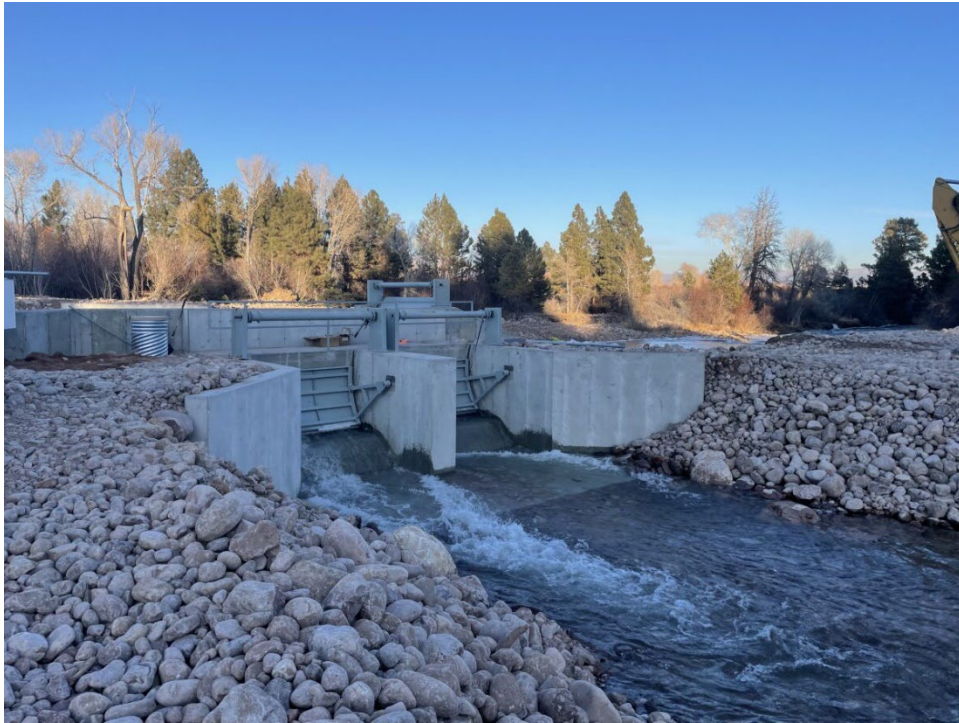
Uintah River bifurcation replacement, Uintah Indian Irrigation Project, Utah – construction complete – radial gates shown are about 4 feet tall.
