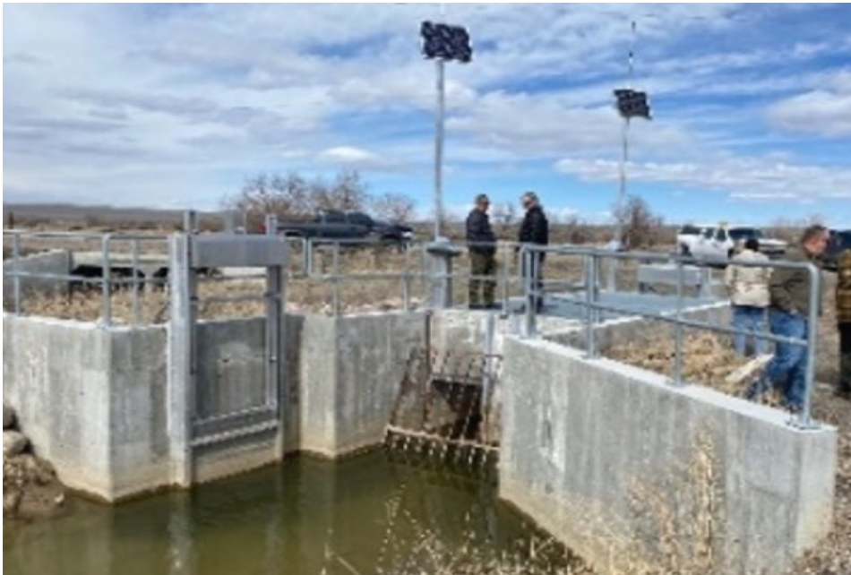
New headgate and turnout at Wind River Indian Irrigation Project
