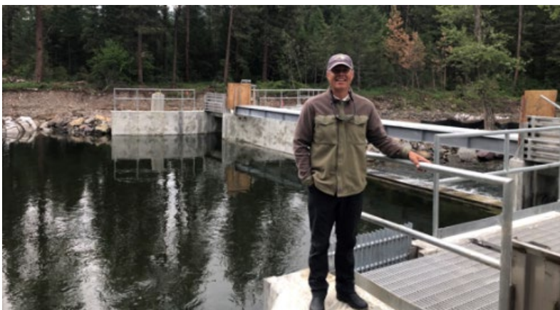
Regional Irrigation Engineer, Dan Lozar, at Jocko K Diversion and Fish Screen at Flathead Indian Irrigation Project, MT
