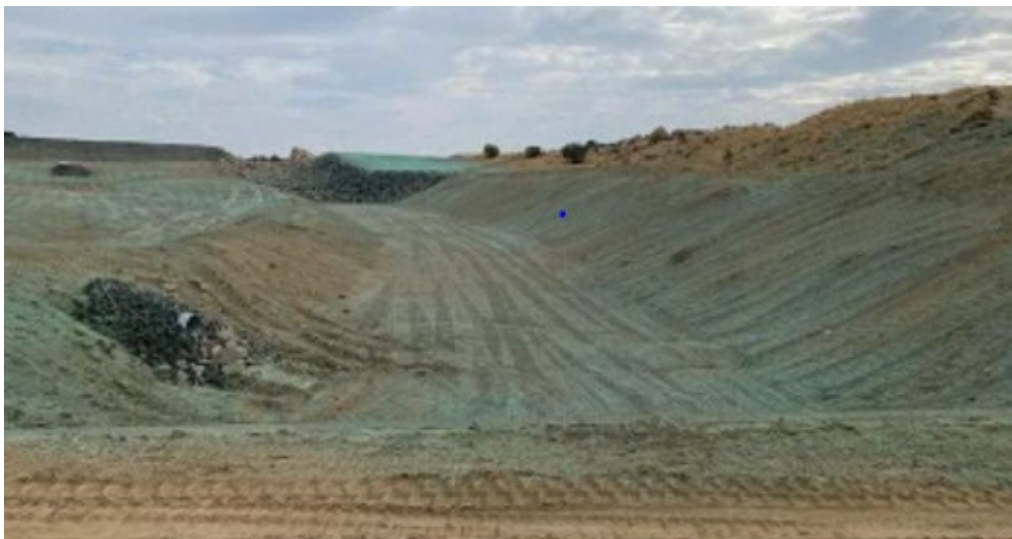
To'hajiilee Dam Spillway, August 2023
