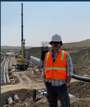
Four Horns Dam Construction
