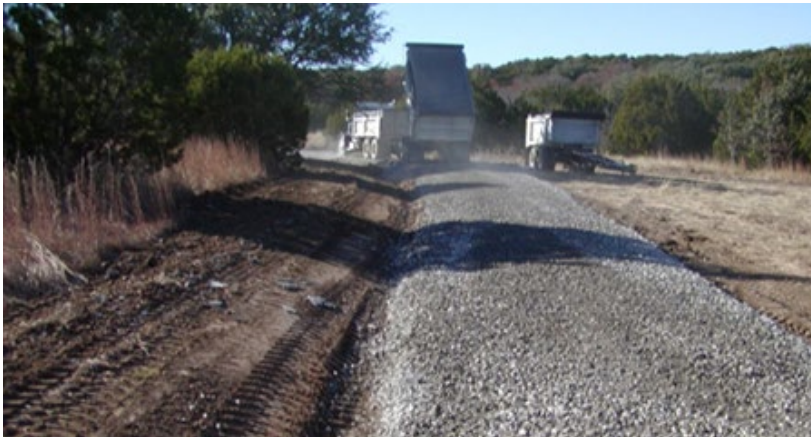
Laying down aggregate road base
