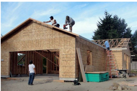
House under construction on Suquamish Indian Reservation
