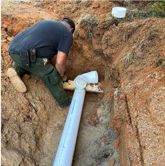
Installation of wet system that conveys harvested rainwater to the storage tank
