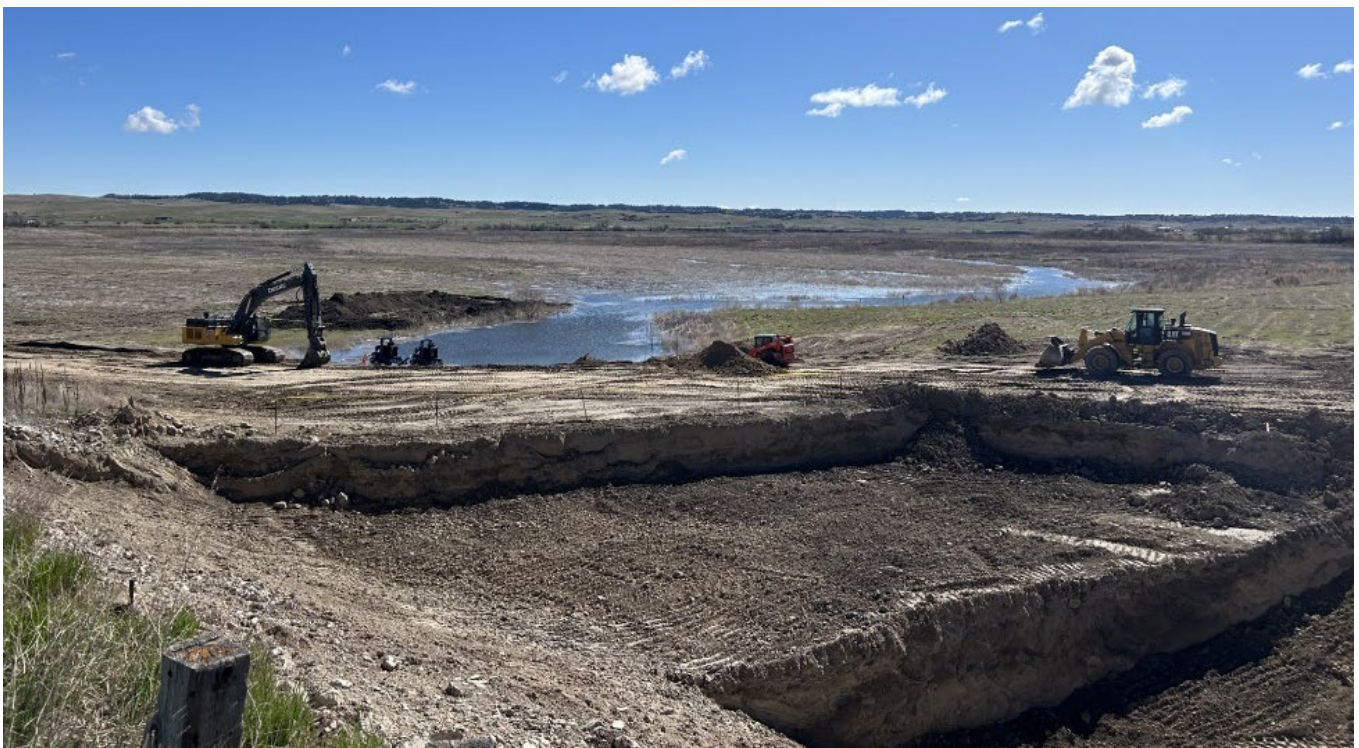
Oglala Dam intake and upstream spillway excavation
