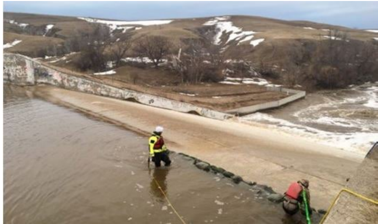
Dam Safety staff sandbagging the Oglala Dam spillway during 2019 flooding
