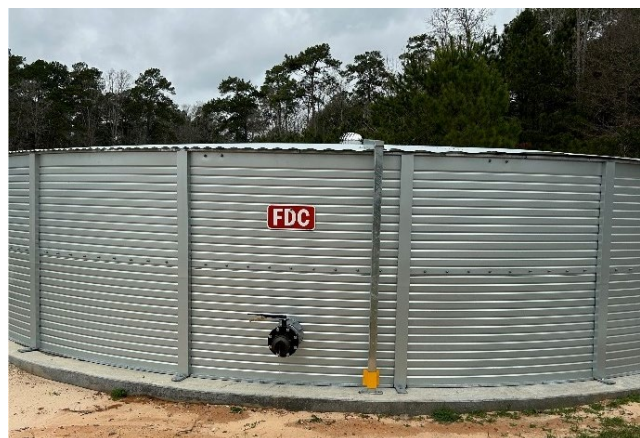
65,000-gallon storage tank
