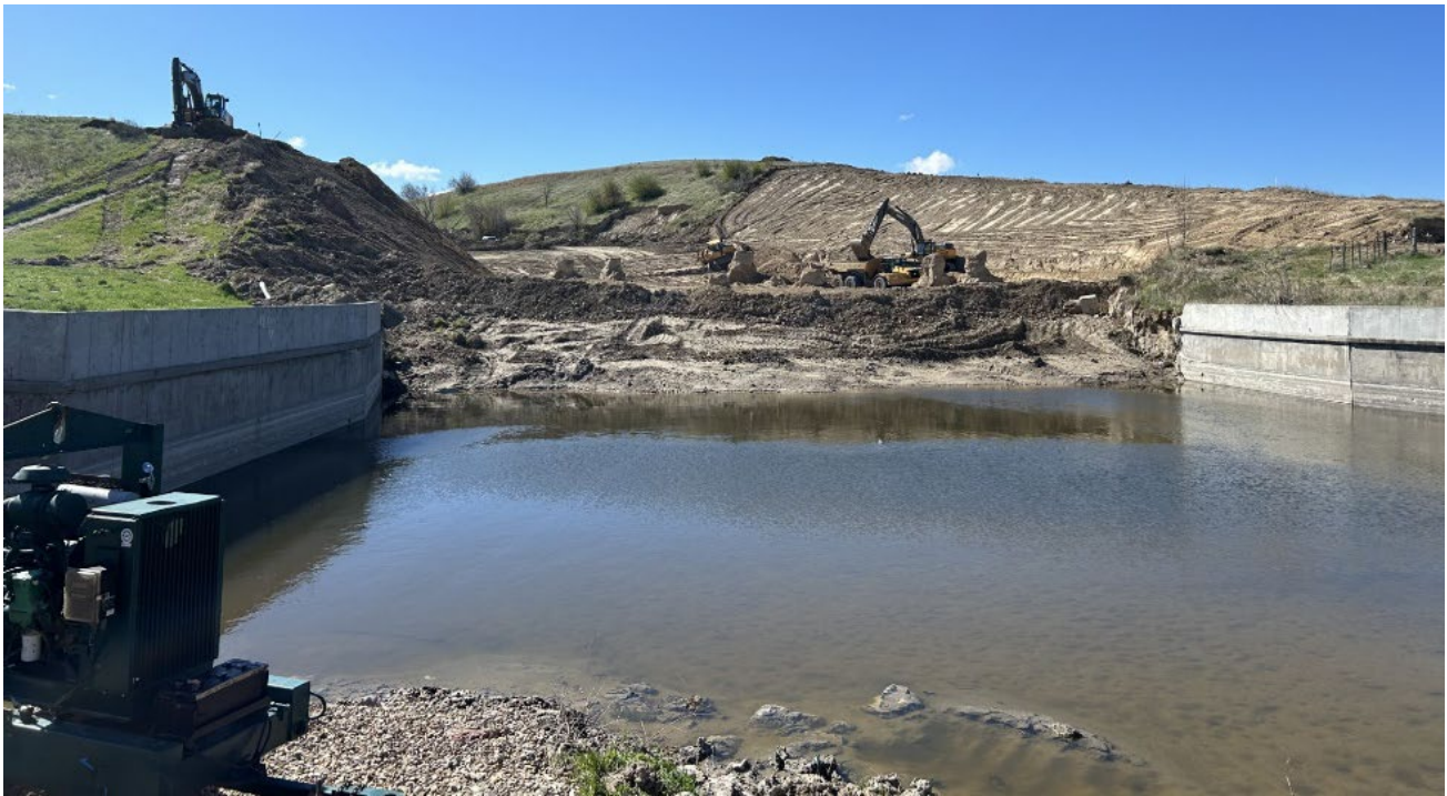
Oglala Dam stilling basin looking upstream to the spillway evacuation
