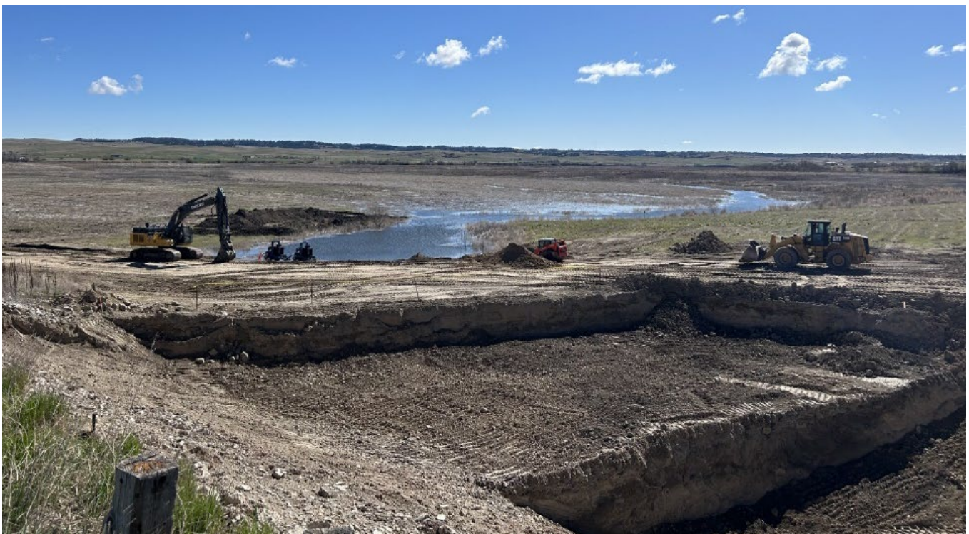
Oglala Dam intake and upstream spillway excavation
