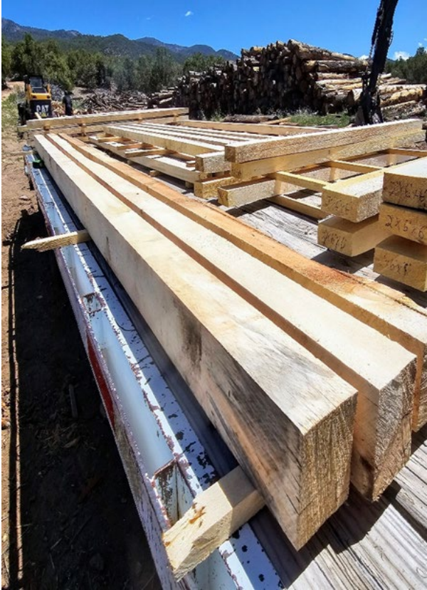
Rough sawn lumber for Tribal construction
