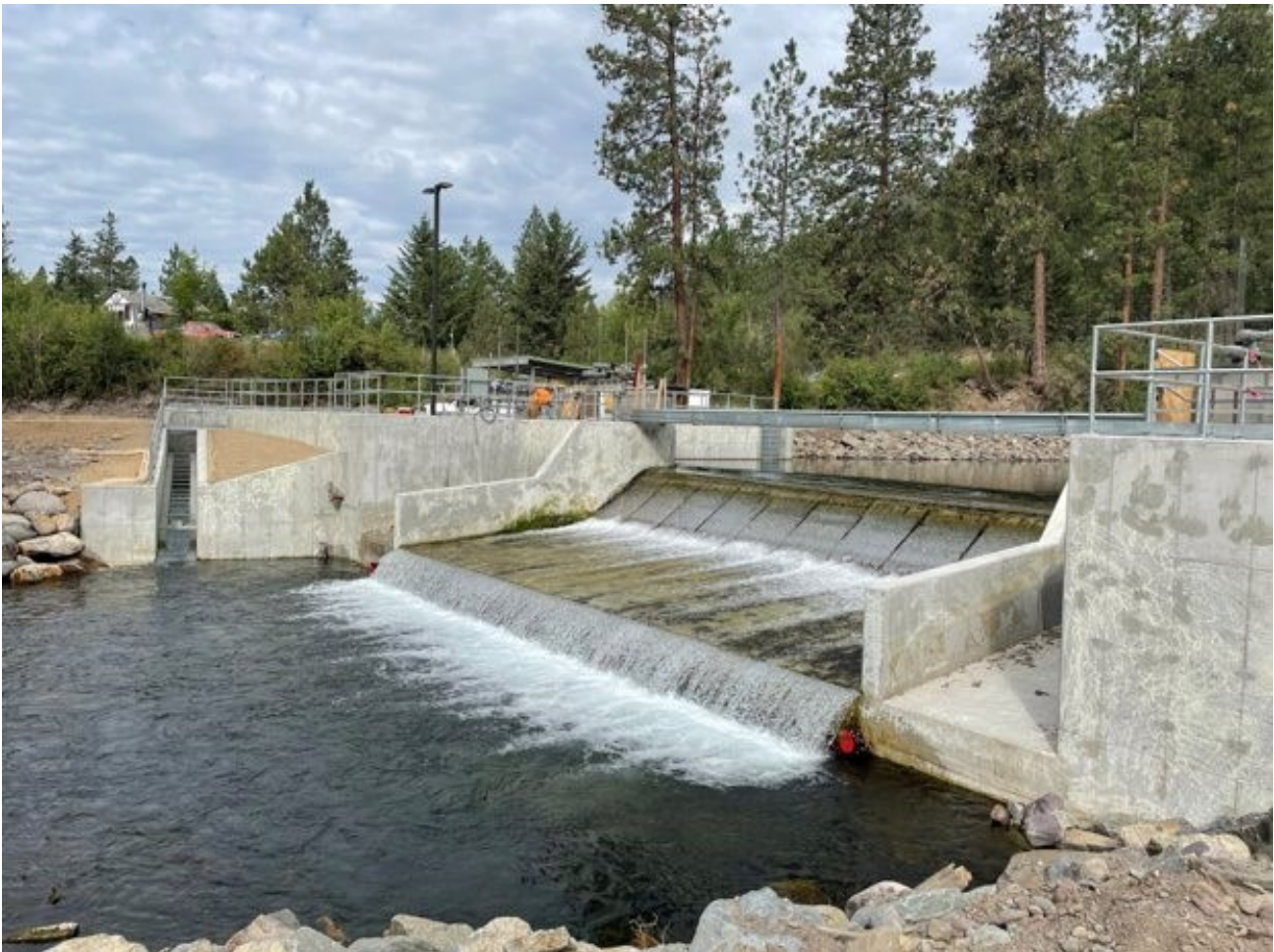
New Jocko Conversion Dam at Flathead Indian Irrigation Project, Montana
