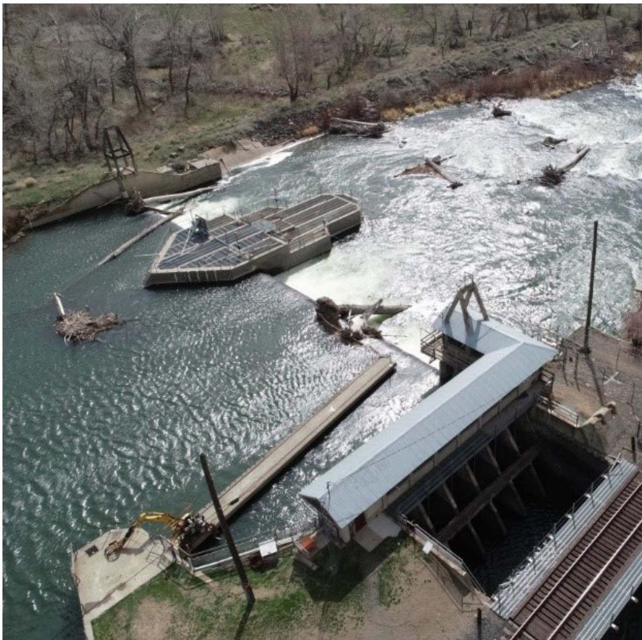
Wapato Diversion at Wapato Irrigation Project, Yakima, Washington
