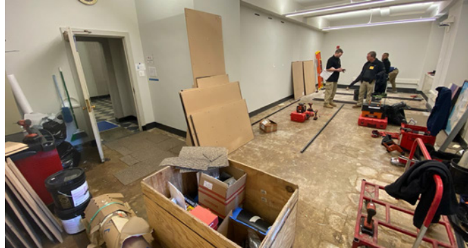
Carpet removed preparing to install rolling racks
