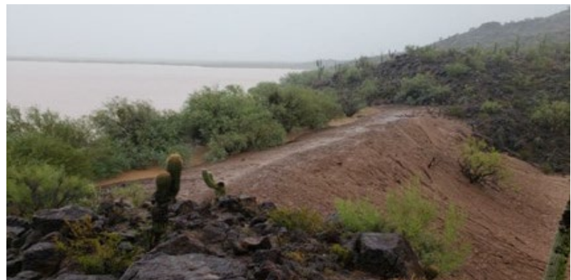
Menager’s Dam during tropical storm Rosa, October 2018
