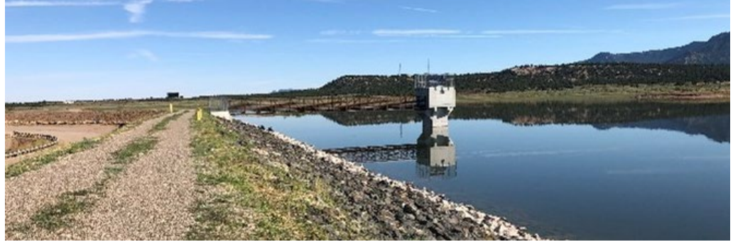
Tufa Stone Dam in San Carlos, AZ
