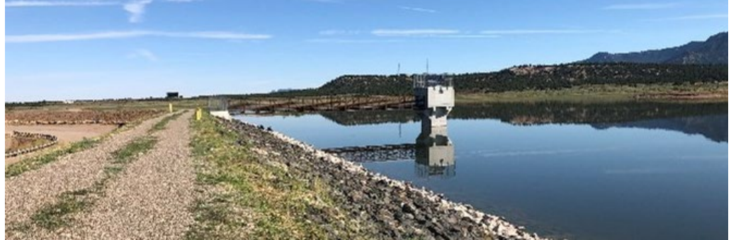
Tufa Stone Dam in San Carlos, AZ
