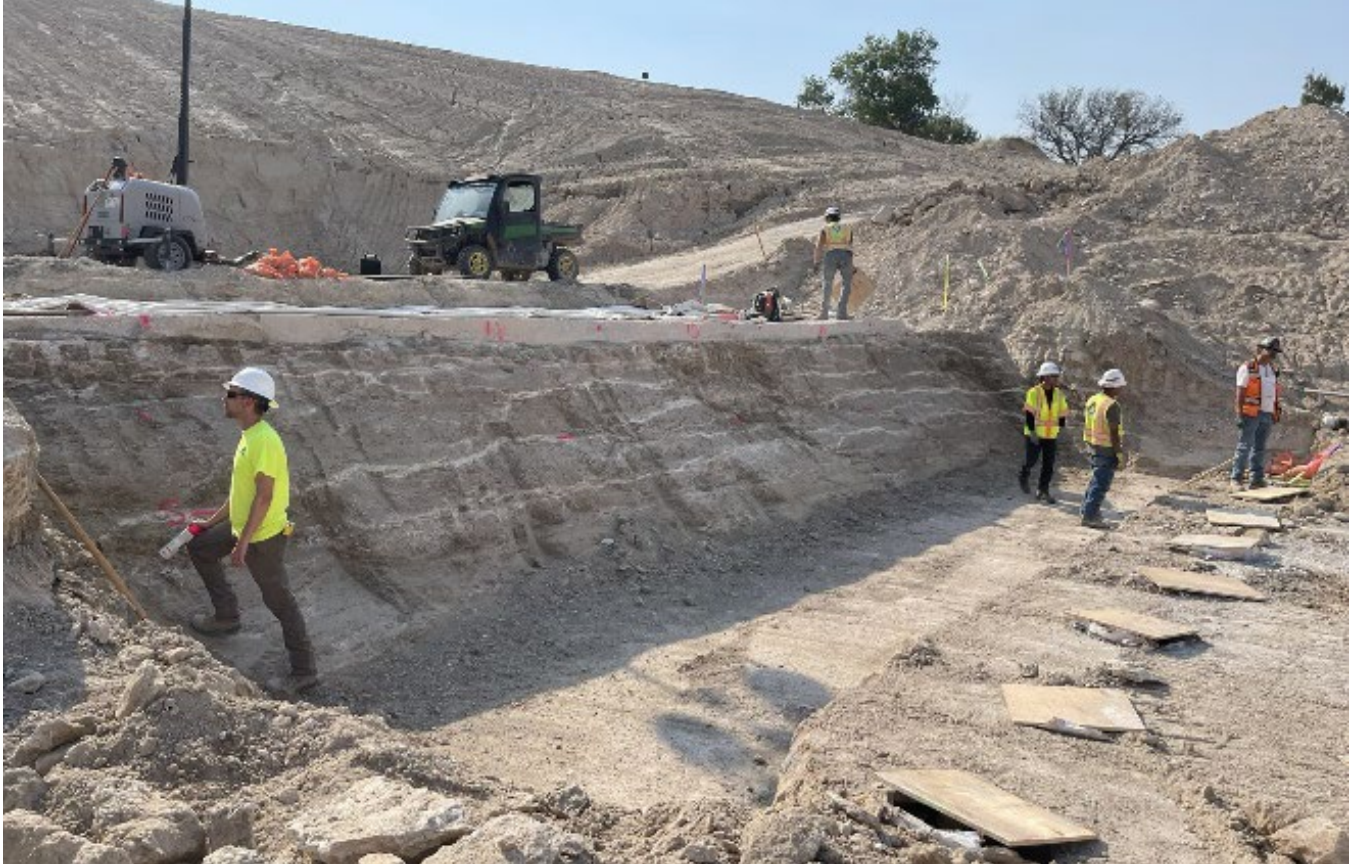
Exposed bedrock near the bottom of the excavation for the new spillway at Oglala Dam; placing the first layer of concrete for the new spillway at Oglala Dam
