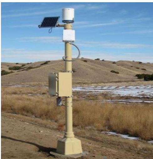
Early Warning System
