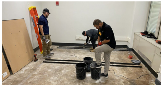
Preparing to install rolling racks, Space Saver cabinets & shelving
