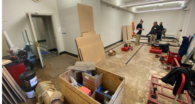
Carpet removed preparing to install rolling racks
