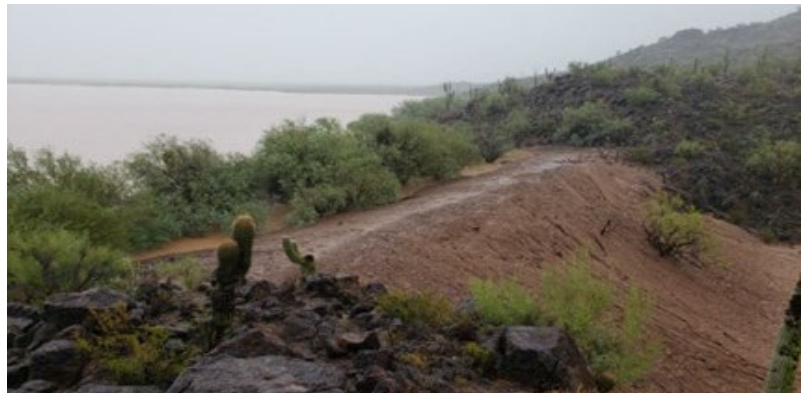
Menager’s Dam during tropical storm Rosa, October 2018
